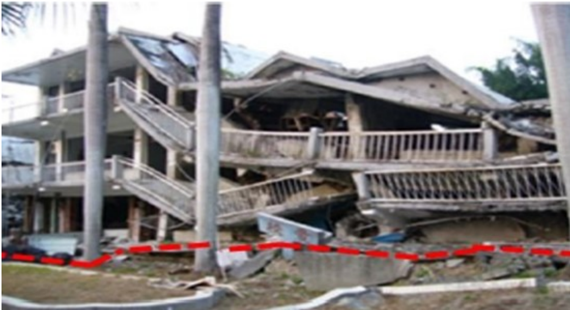
Figure 7. Collapse of Guangfu Junior High School in Taichung, Taiwan during the 921 Jiji earthquake in 1999 (Hsu, 2022).
